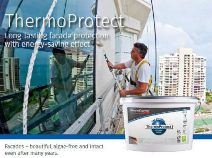
The ready-to-use facade coating protects against weathering, algae, moss and fungal growth and improves the year-round energy balance of the building. ThermoProtect is a facade paint and high-quality dispersion that keeps the facade dry, regulates moisture and temperature and is exceptionally robust and durable.
