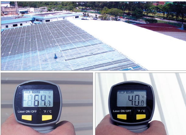
Industriehalle in Malaysia.
