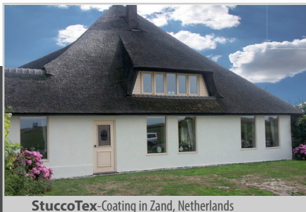
StuccoTex-Coating in Zand, Netherlands
