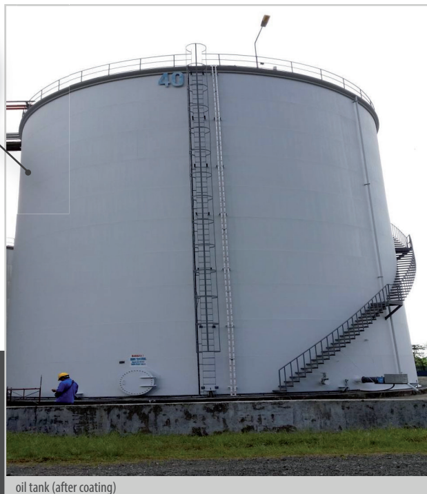
oil tank (after coating)
