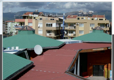
ThermoActive-coating in Izmir, Turkey
