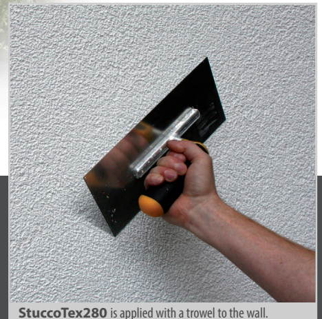
StuccoTex280 is applied with a trowel to the wall.
