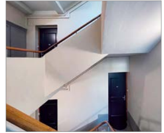
... and stairwells (FR).
