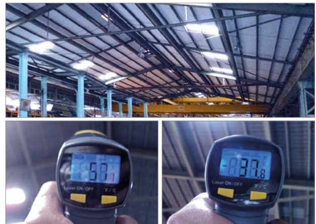
Hall roof inside (before-after): The temperature was reduced by 19.3°C. Use: Improved working conditions, energy saving, cost reduction of roof maintenance.
