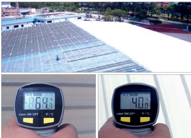
Industrial hall in Malaysia. Hall roof outside (before-after): The roof coating reduced the surface temperature by 24.7°C.
